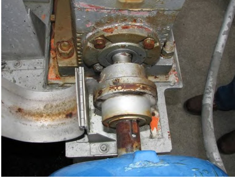
Figure 16-2. Gear Coupling with Grease Fitting.
